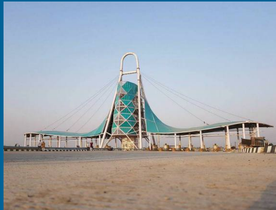
KUNDALI TOLL PLAZA, EASTERN PERIPHERAL EXPRESSWAY
