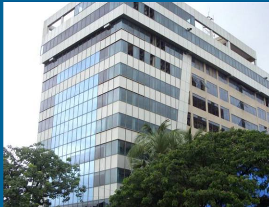
SOLARIS COMMERCIAL BUILDING
